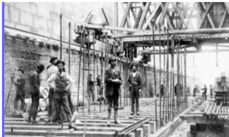
Construction of the Sault Ste. Marie Canal, November 1893
